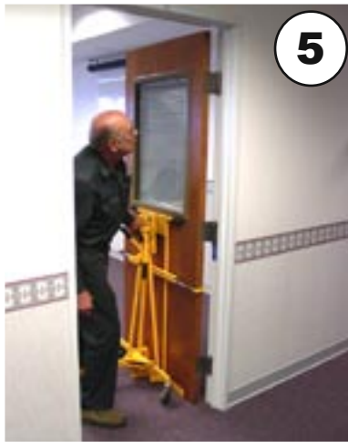
Adjust Doorminator™ so that the door is parallel with the jamb and hinges align.
